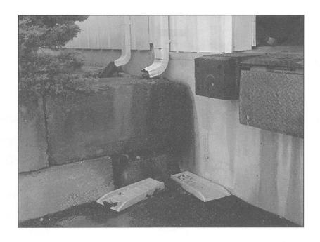
With a small modification of a gutter spout and an expense of less than \$100, Lampin Corporation will prevent more than 73,000 gallons of stormwater runoff per year.
